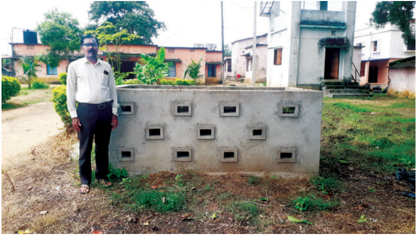
NADEP Compost Pit
